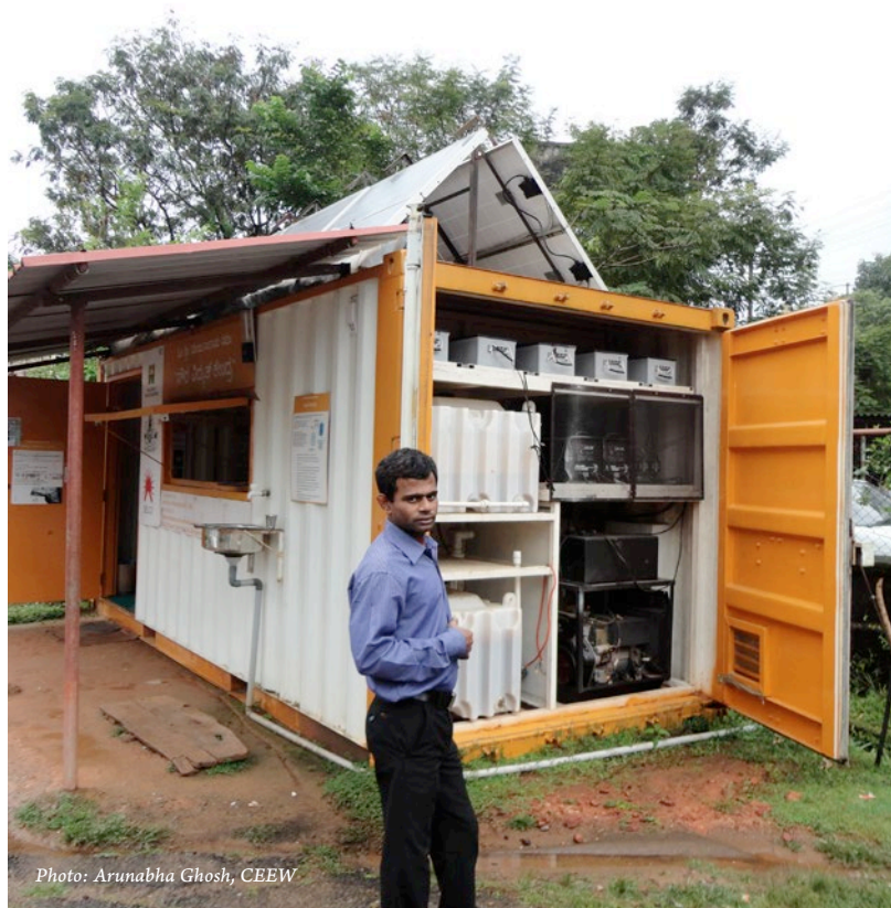
Operator of a solar kiosk stands outside the kiosk converted from a shipping container (water tanks and inverters visible), Dharmasthala Village, Dakshin Kannada District, Karnataka
