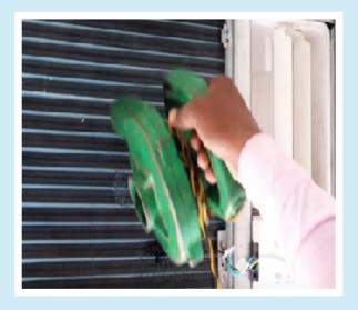
In addition to the above, at least once a year, a proper cleaning agent should be used to clean the condenser coil.
