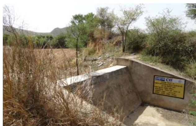
Figure 19: Check dam built by the project team in Neemrana
