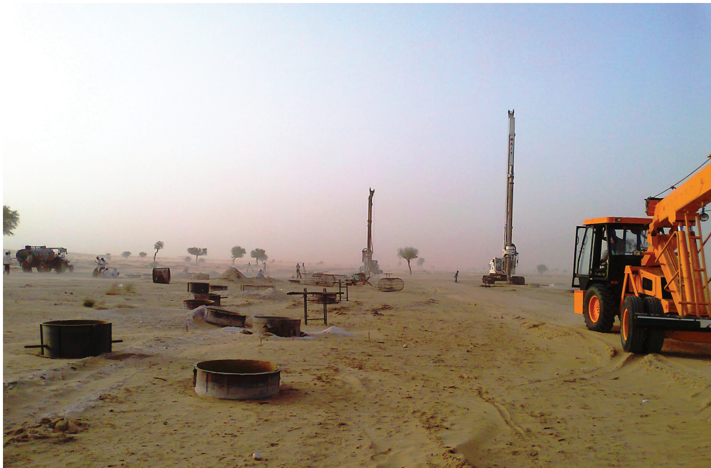
Grid-connected CSP project currently being constructed under the NSM. Photo used with permission.
