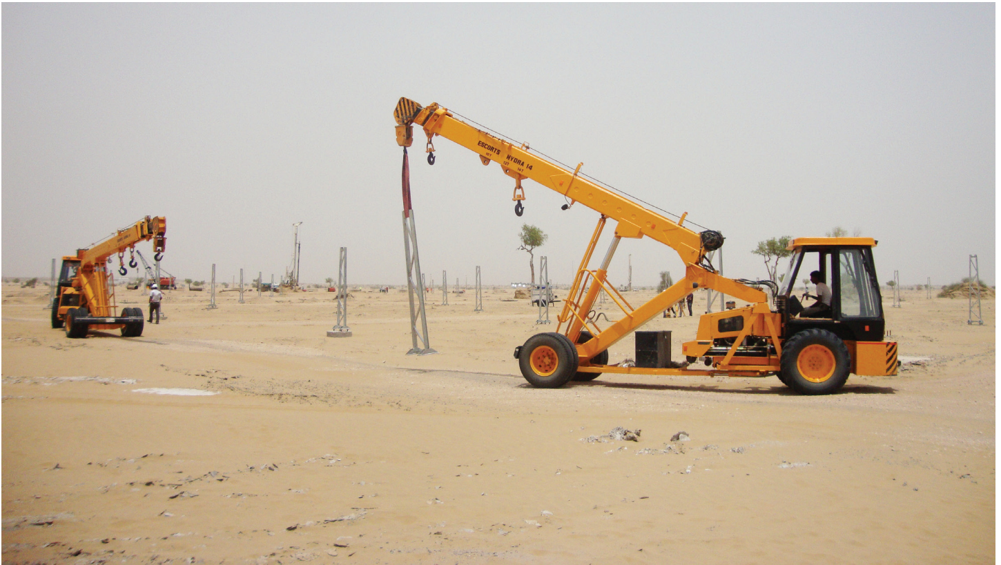
Grid-connected CSP project currently being constructed under the NSM. Photo used with permission.
