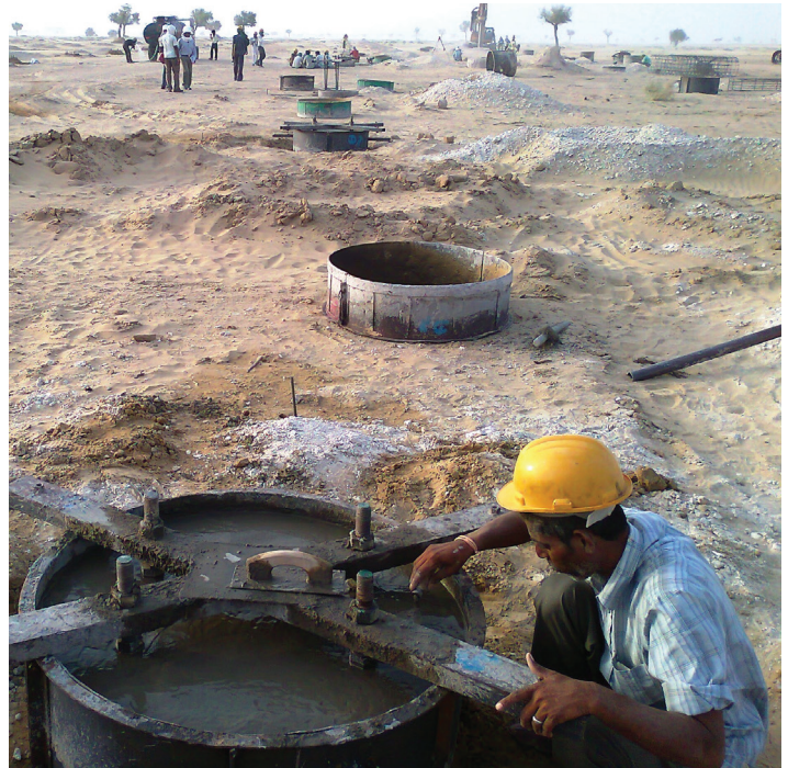
Grid-connected CSP project currently being constructed under the NSM. Photo used with permission.
