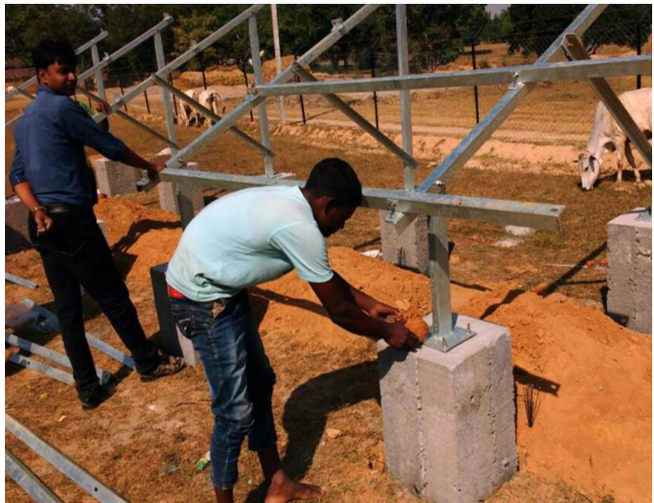
Local workers installing the framing for photovoltaic (PV) solar panels
