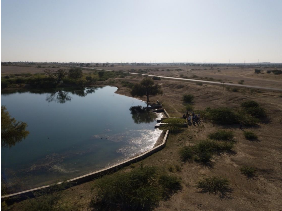
Image 3: Rainwater harvesting structure ‘khadin’
