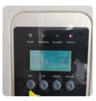
Non functioning inverter due to any internal cause resulting in system shutdown and no energy output
