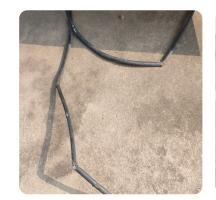
**Damaged cable** due to improper maintenance causing high resistance and safety concerns **Possible causes** improper structure for wiring, reckless activity near the wires
