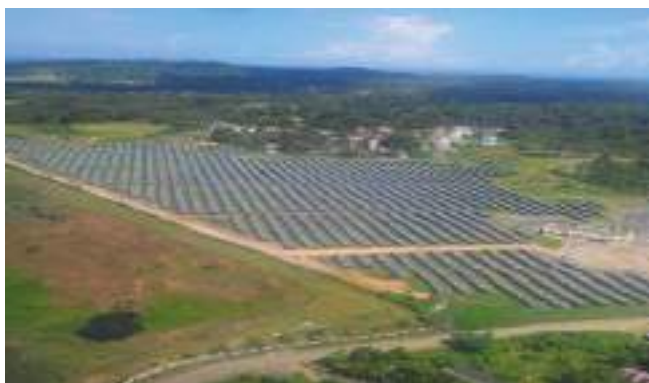
Figure 6.6: 5 MWp Solar PV Plant commissioned at Garcharma, Port Blair, Andaman & Nicobar islands
