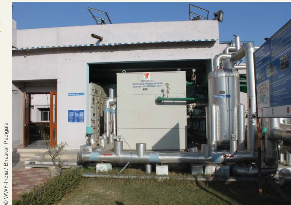
FIGURE 2.9 Triple-Effect Absorption System Installed at the Solar Energy Center (SEC)
