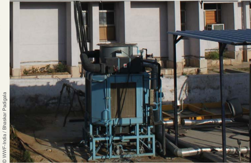
FIGURE 2.20 Double-Effect Vapour Absorption Chiller (15kW) at SEC, Gurgaon
