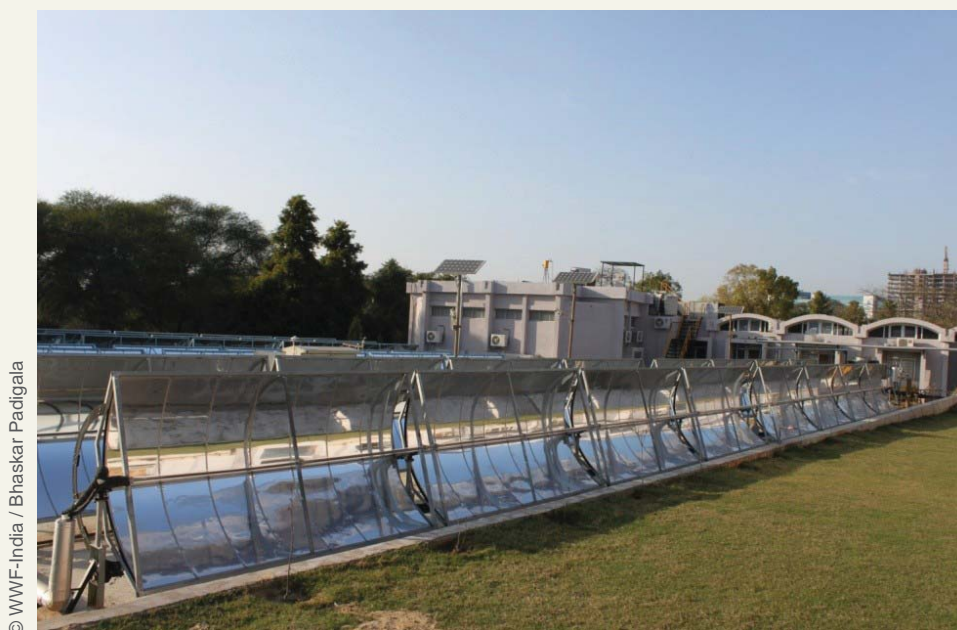
FIGURE 2.19 PTC-Based Solar Air-Conditioning System at SEC, Gurgaon
