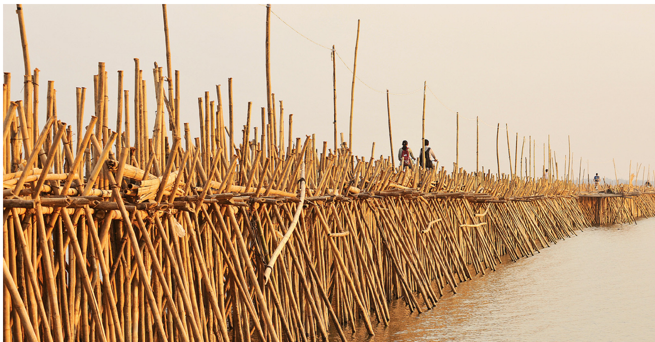
The 3,000-foot Bamboo Bridge on the Mekong River, Kampong Cham, Cambodia, is one of the world's longest bamboo bridges. The bridge, a green infrastructure-based NbS solution, ensures connectivity for locals and tourists by adapting to seasonal water level changes.
