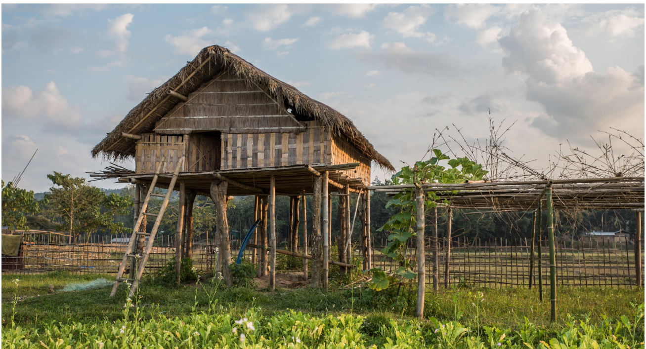
Traditional stilt houses made of local material are local NbS that can protect against floods. This is a stilt bamboo house in the Dispur district of Assam, one of India's most flood-prone states.
