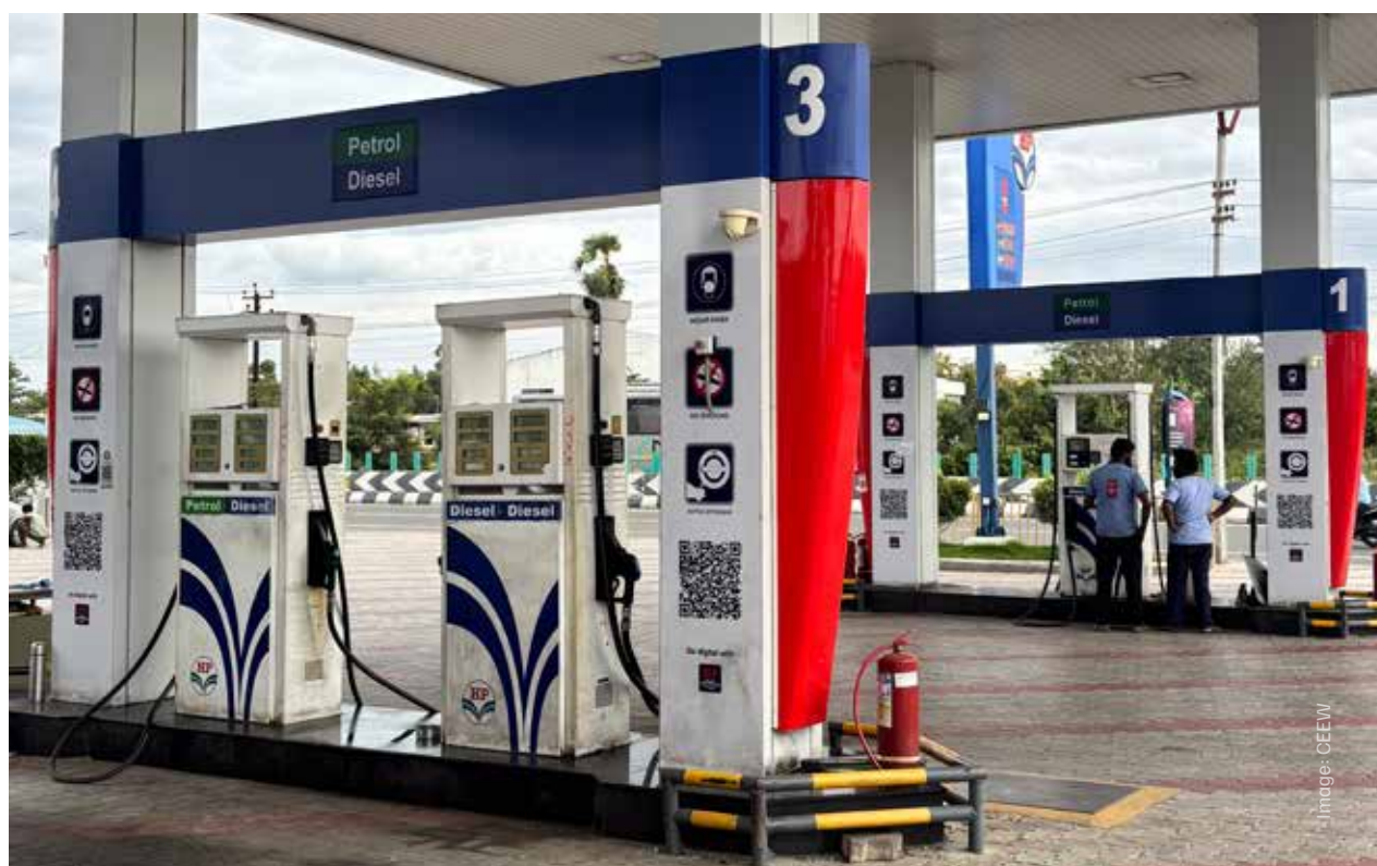
Petrol pumps in Erode
