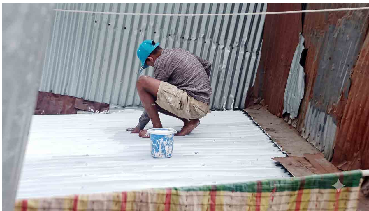
A local painter applies cool roof coating on a corrugated-iron roof in Karail slum, Dhaka.
