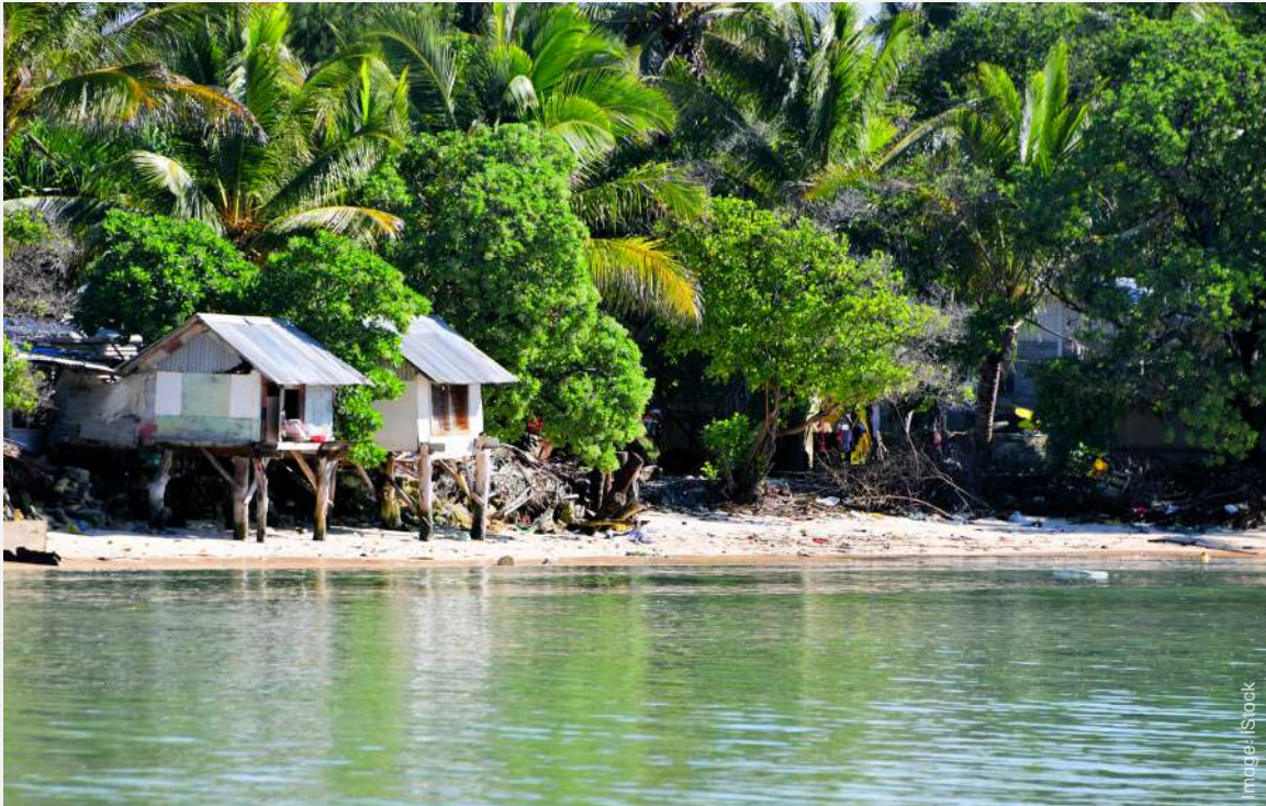
Houses on stilts built by communities in low-lying areas to overcome coastal flooding, high tides and rising sea level.
