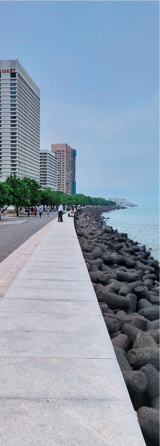
Climate-resilient urban infrastructure: The tetrapod seawall along Marine Drive, Mumbai
