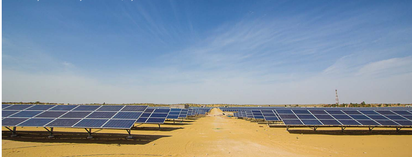
NSM Utility Scale Solar Project in Jaisalmer, Rajasthan
