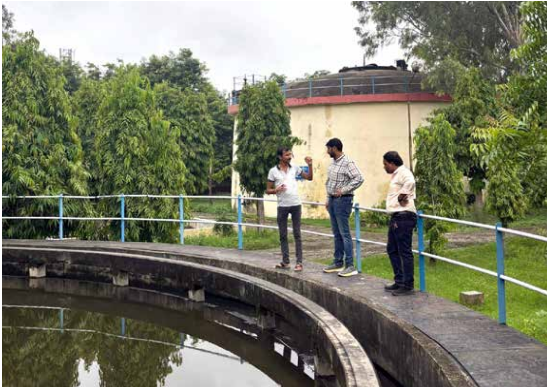
b) CEEW team's visit to the Banaras Locomotive Works sewage treatment plant of 12 MLD capacity
