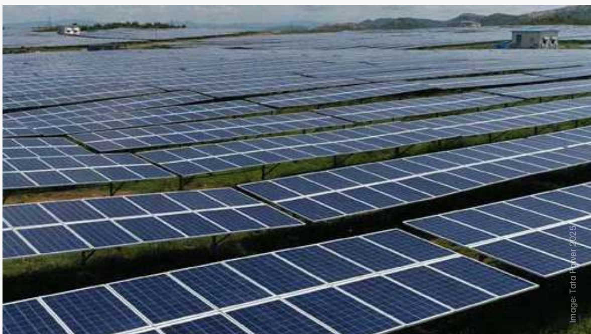
Tata Power’s terrain tracking solar plant resulting in reduced ecological impacts.
