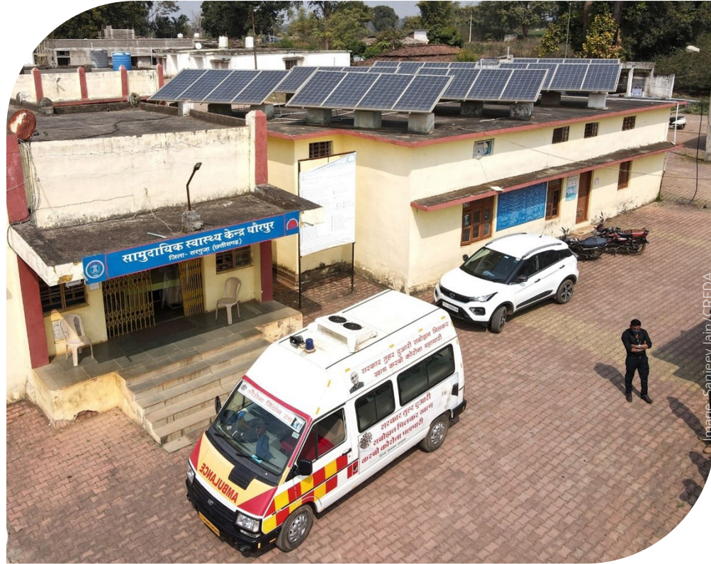
A solar-powered primary health care centre in Chhattisgarh, India.
