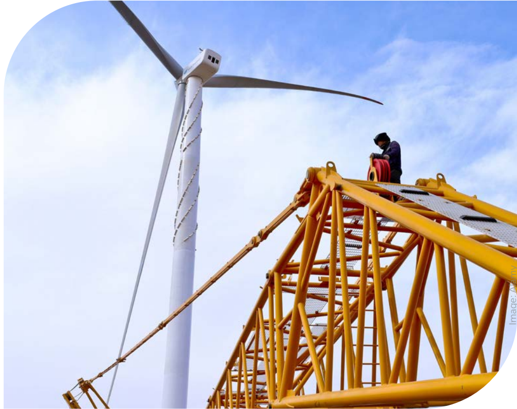
Setting up wind turbines in China.
