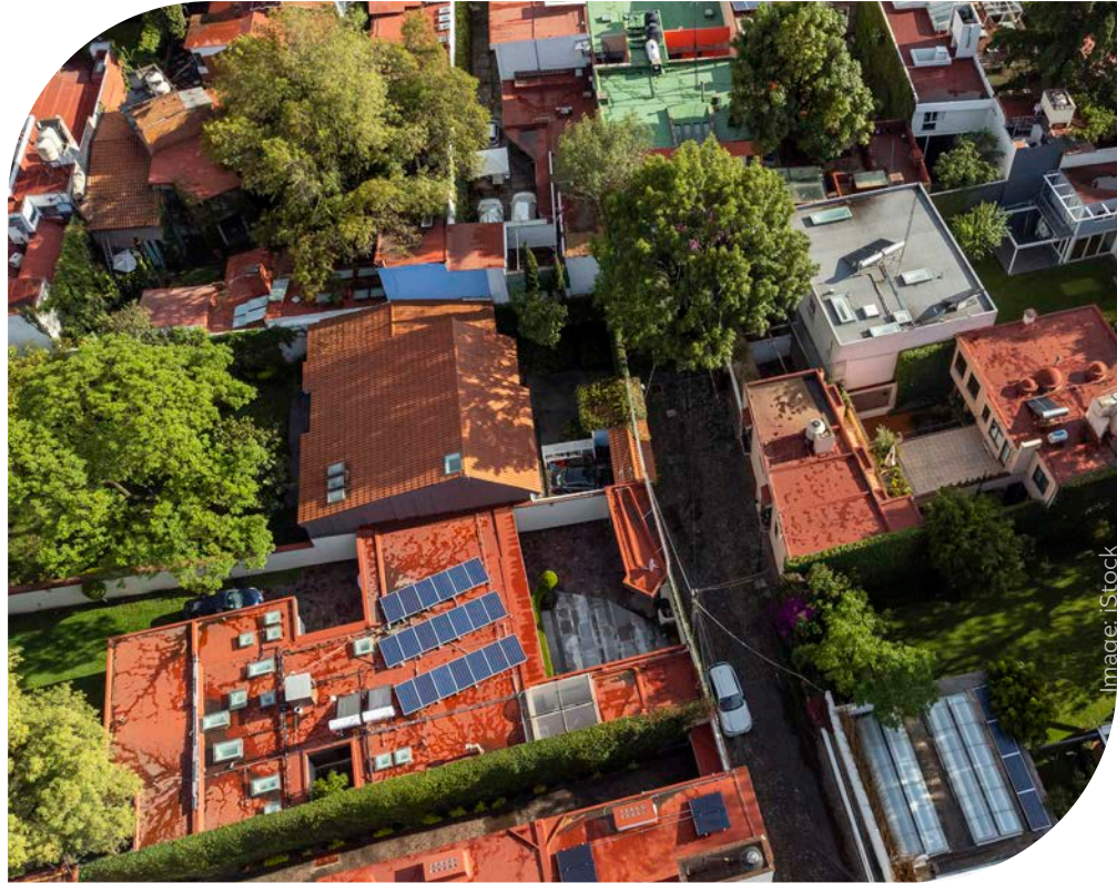
Rooftop solar in Mexico
