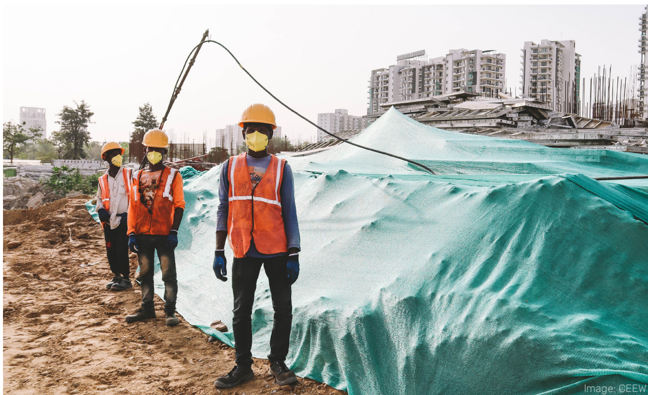
Proper covering of loose soil and debris is crucial to ensuring worker safety, reducing dust pollution, and preventing accidents at construction sites.
