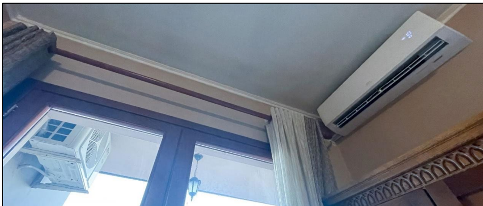
Figure 3: Domestic AC/HP in use. The system consists of an outdoor unit and an indoor unit connected by piping
